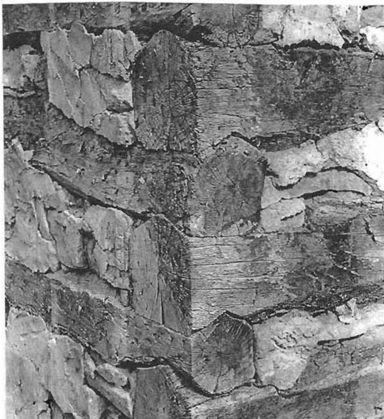
Figure 5: "V" notching of the corner log joints and chinking (pg 11).
