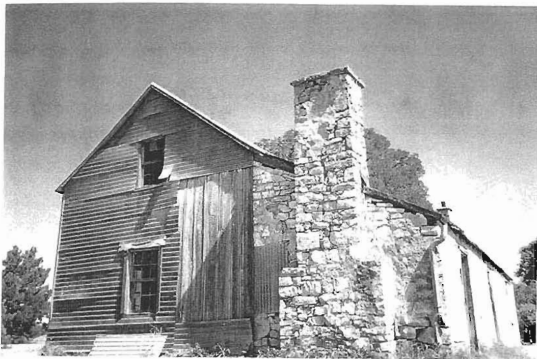
Figure 9: Tin siding on top of cut board siding. Logs are beneath the boards (pg 13).
