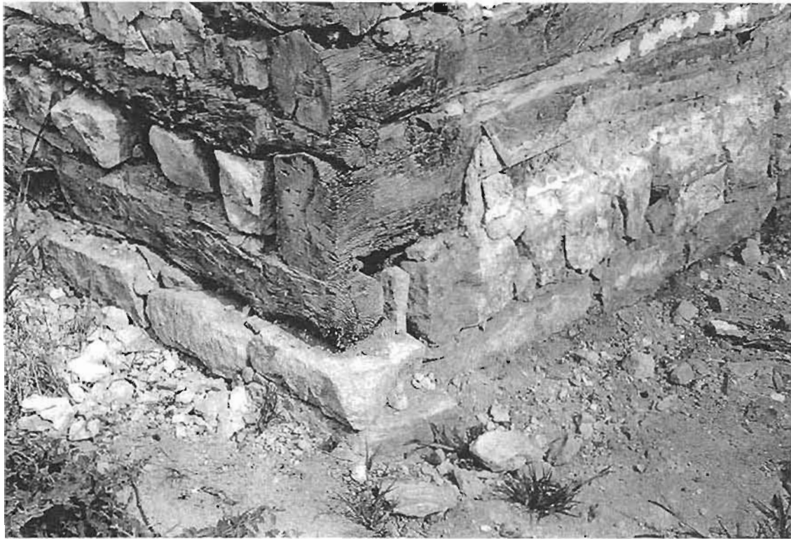
Figure 7: Stone footing supporting the log walls (pg 12).
