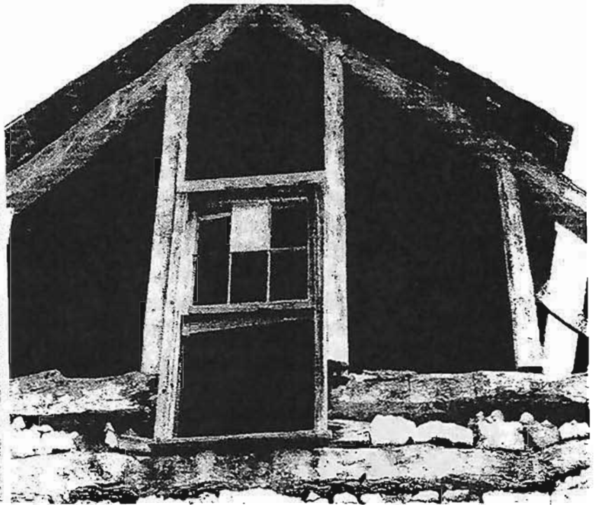
Figure 6: Inside of roof with no ridge pole.
