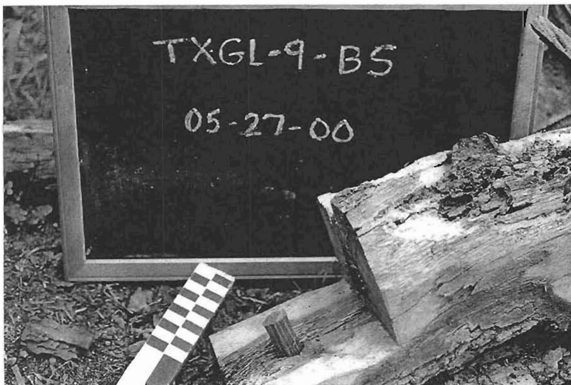
Figure 10: Pegs used to hold door jam logs together (pg 14).
