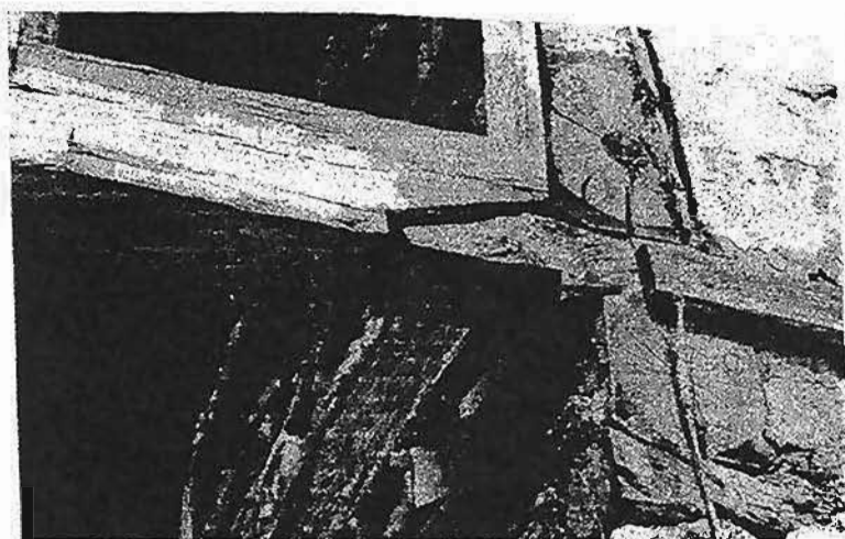
Figure 13: Joint on the cantilevered portion of the second story floor joist.
