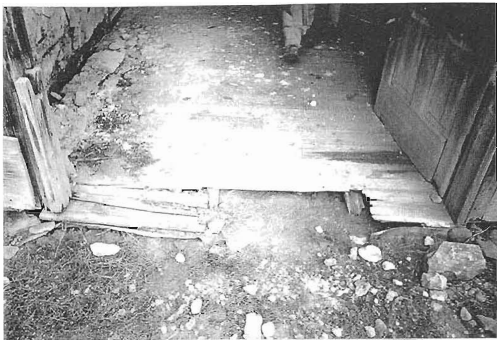
Figure 8: Floor joist protruding from flooring (pg 13).
